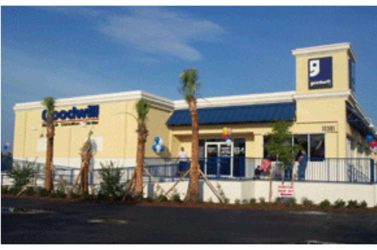
Punta Gorda store located at 10381 Tamiami Trail.
